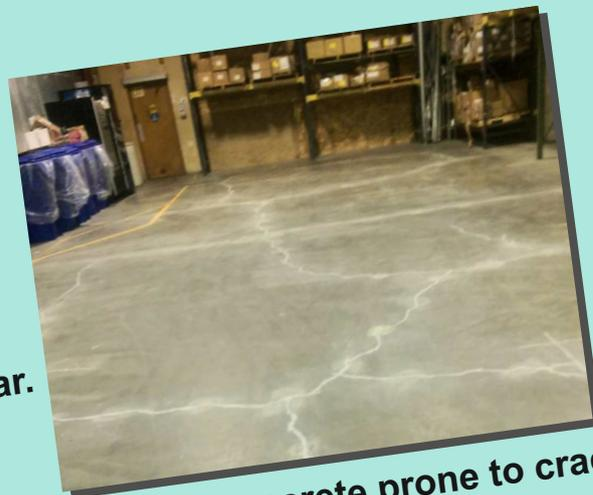
Conventional concrete prone to cracking.
